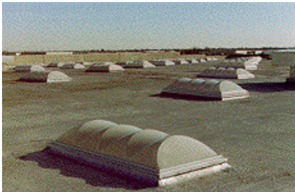
Figure 8: Compound parabolic skylight
